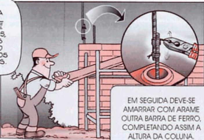
EM SEGUIDA DEVE-SE AMARRAR COM ARAME OUTRA BARRA DE FERRO, COMPLETANDO ASSIM A ALTURA DA COLUNA.
